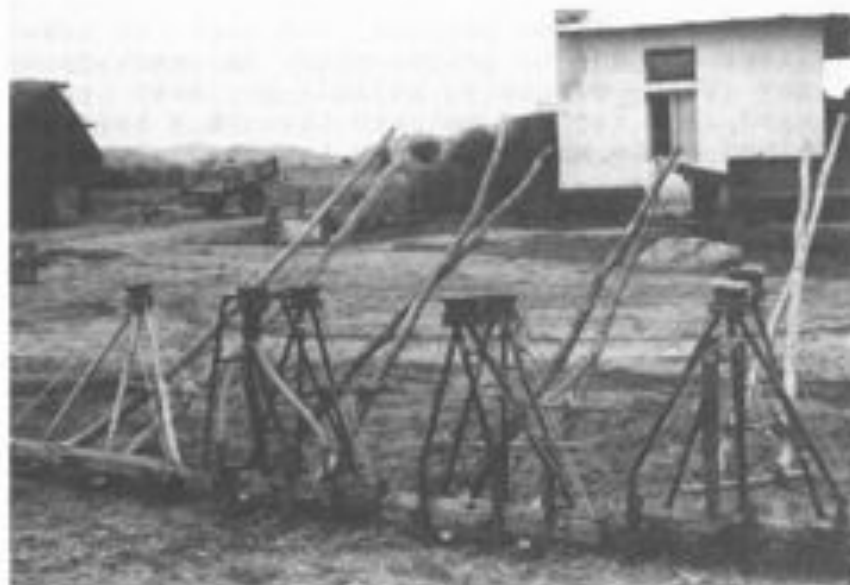
Figure 6.7 Three Row Hand Drilling Equipment. (Tippen)
