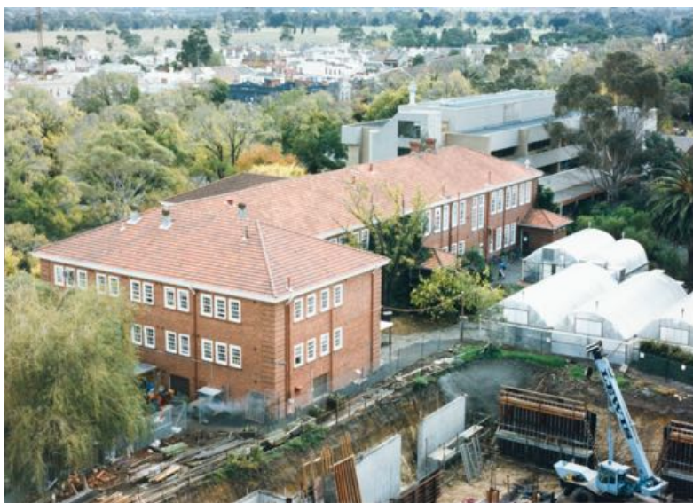
Old Agriculture: Greenhouses in System Garden for Construction of Zoology, 1986 184
